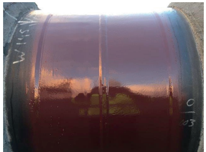
Figure 3. Coating external field joints assures seamless corrosion prevention.
