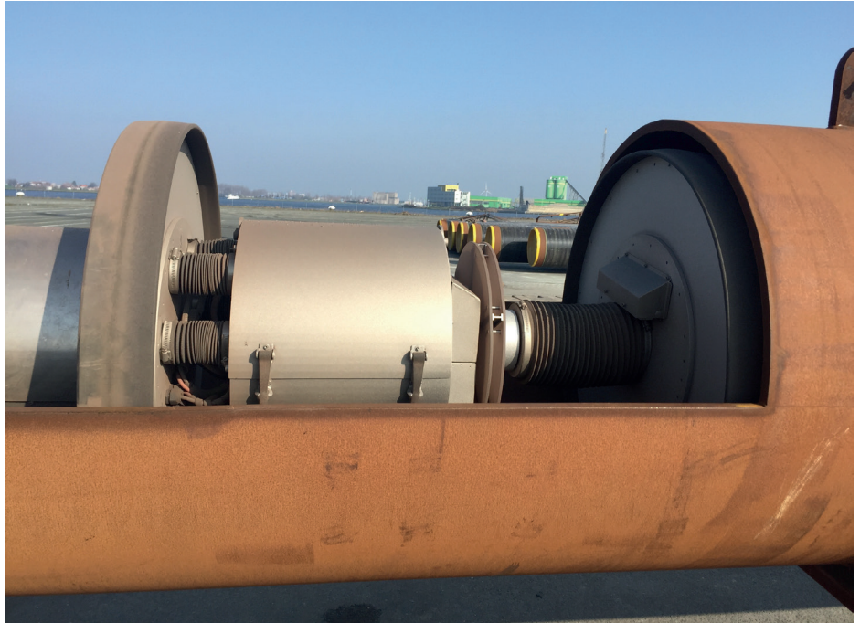
Figure 2. The robotic cleaner ensures a surface profile that the coating will adhere to, providing seamless corrosion prevention.
